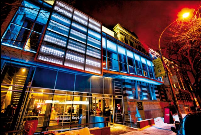
A dynamic lighting scheme of pre-programmed sequences can change the ambience of the Cinémathèque Québécoise.
